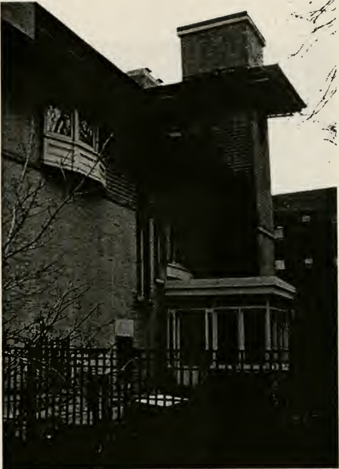
Figure 1.12 Heller House, north façade. Porch and elevator shaft are visible. Photograph by the author, 1999.
